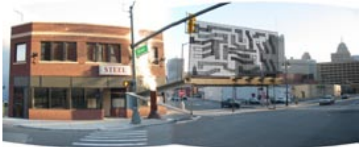
gratiot steam pipe site (right) studies for gateway over the street, and kinds of screens.
