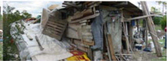
ramp leading to roof
